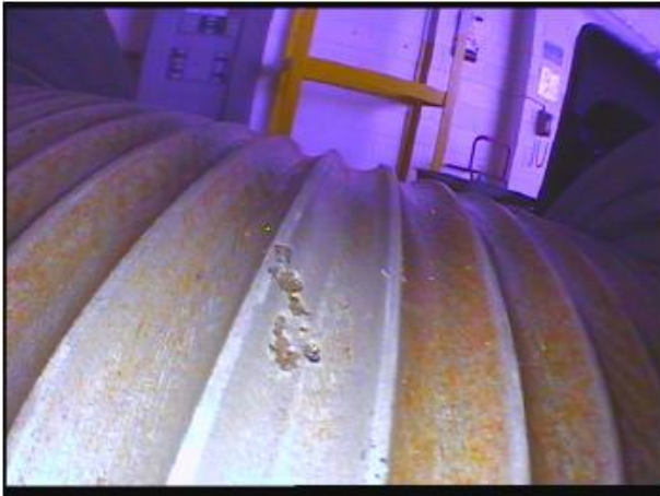
Unacceptable rust and corrosion
