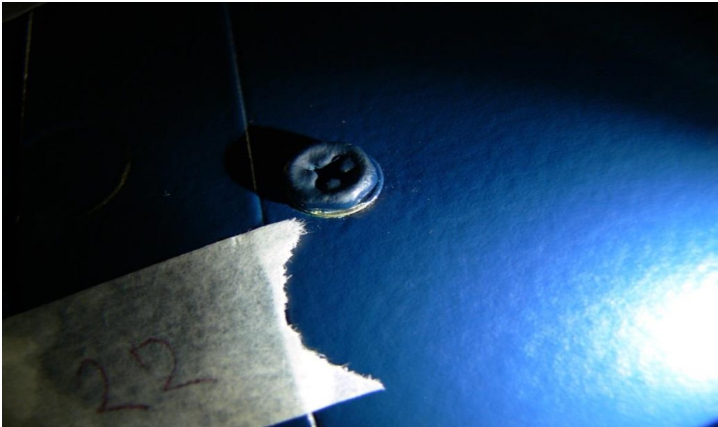
Apply touch up on the bare surface
